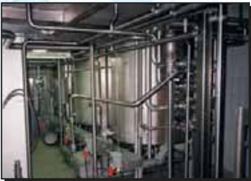
Leveltransmitters on CIP tanks
