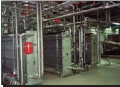
Pressure transmitter on line
